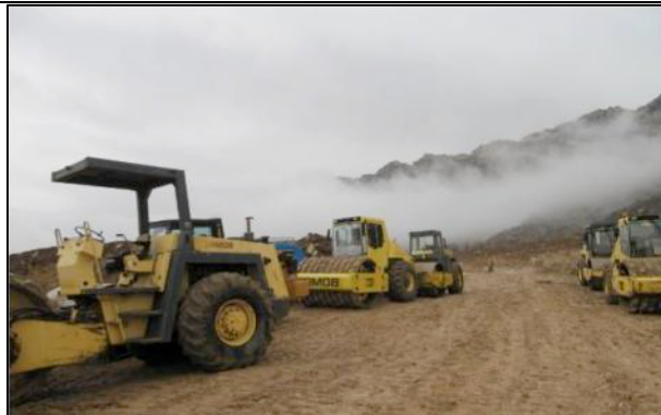
Construction equipment at QD-1, Kurdistan, Iraq 2010
