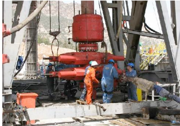
Installing BOP, QD-1 well site, Kurdistan, Iraq, 2010.
